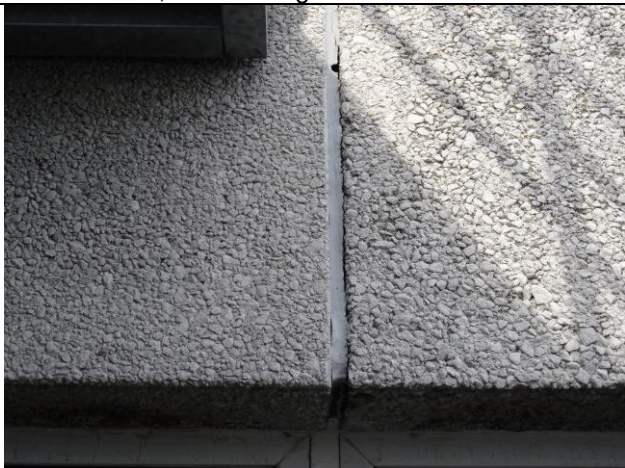
Foto 12: Defekte facadefuger.
